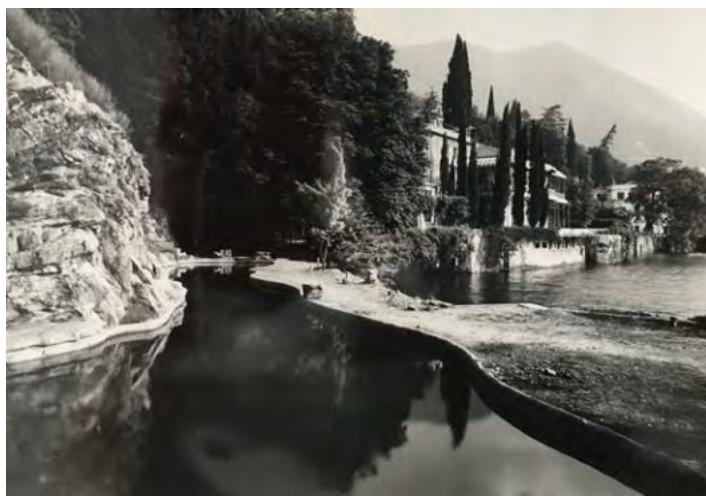
6. The swimming pool under construction, Villa Rospini, Blevio (c. 1955) (Courtesy Renato Wild Archive)
